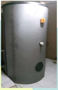
The second centralized SHW system operates similarly with 1 array of 30 tubes and 300l storage tank, dedicated to the kitchen and bar.
